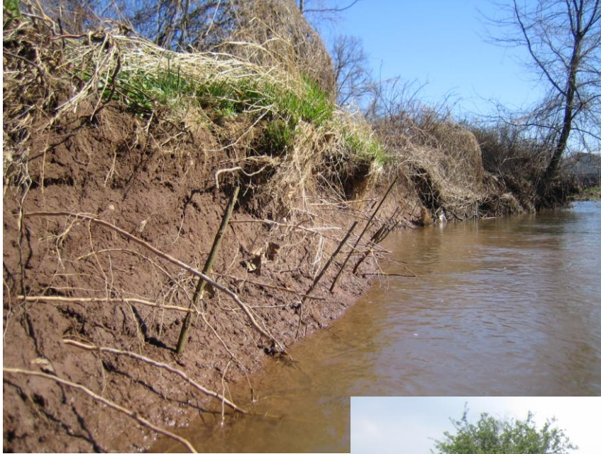
In order to stabilize eroded stream banks, TCCCA volunteers installed black willow live stakes at the Hess farm along the Little Conewago Creek. A year and a half after installation, many of the stakes have taken root and are helping to minimize bank erosion.
